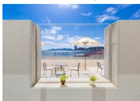
景観配慮型防潮壁 (SEAWALL)
