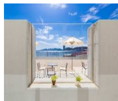
景観配慮型防潮壁 (SEAWALL)
